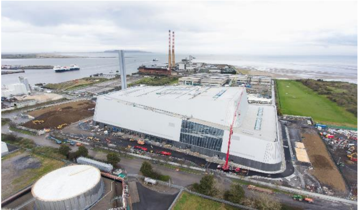
Site Aerial View Looking East March 2017 (Copyright PML).
